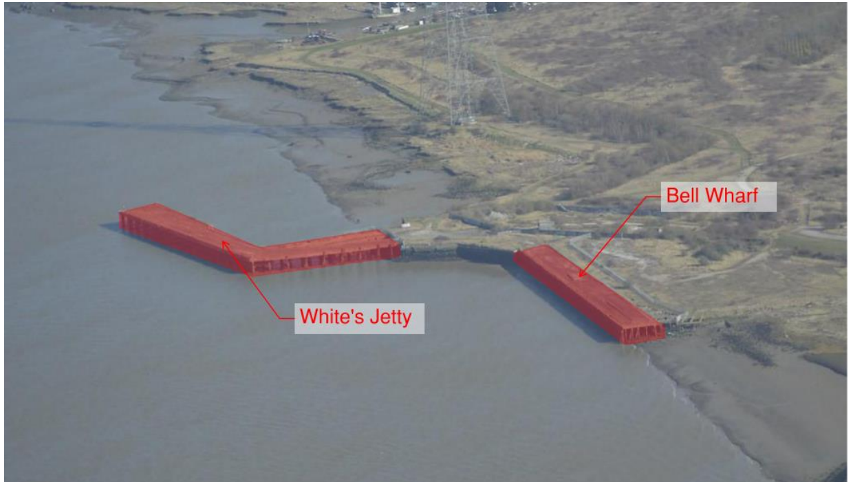
Figure 17.6: Bell Wharf and White's Jetty.
